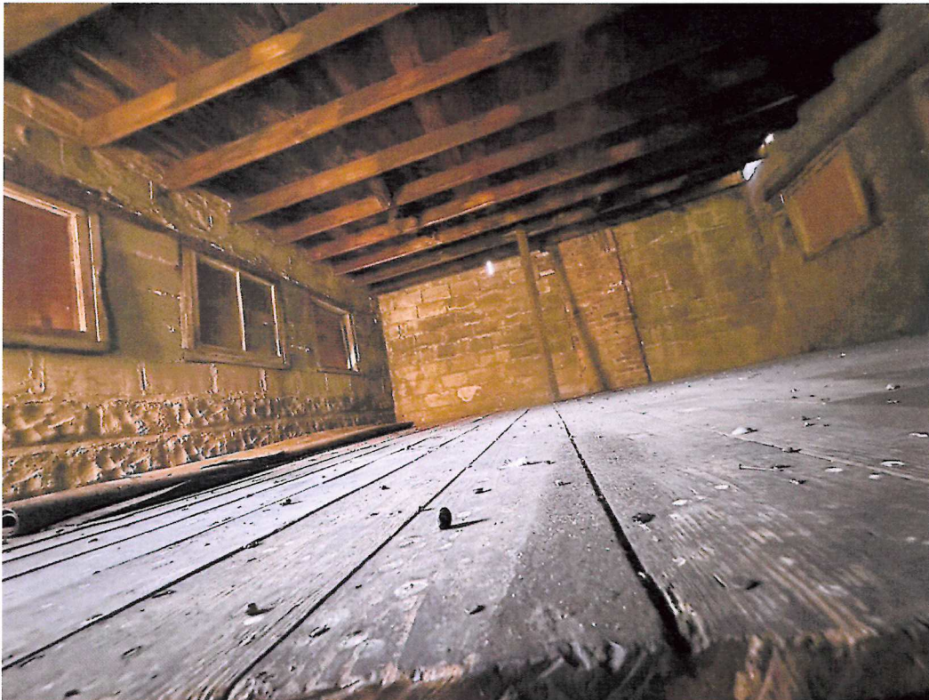
Fourth floor attic space – note combination of brick and CMU construction
