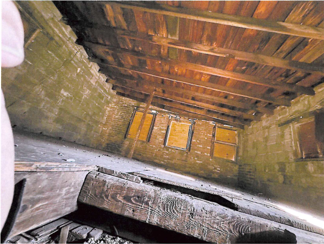
Fourth floor attic space – note combination of brick and CMU construction
