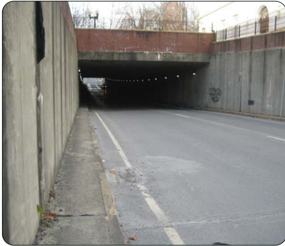
Photo 3: View west toward tunnel. Road shoulder is extremely narrow. Traffic noise in tunnel is very highly amplified.
