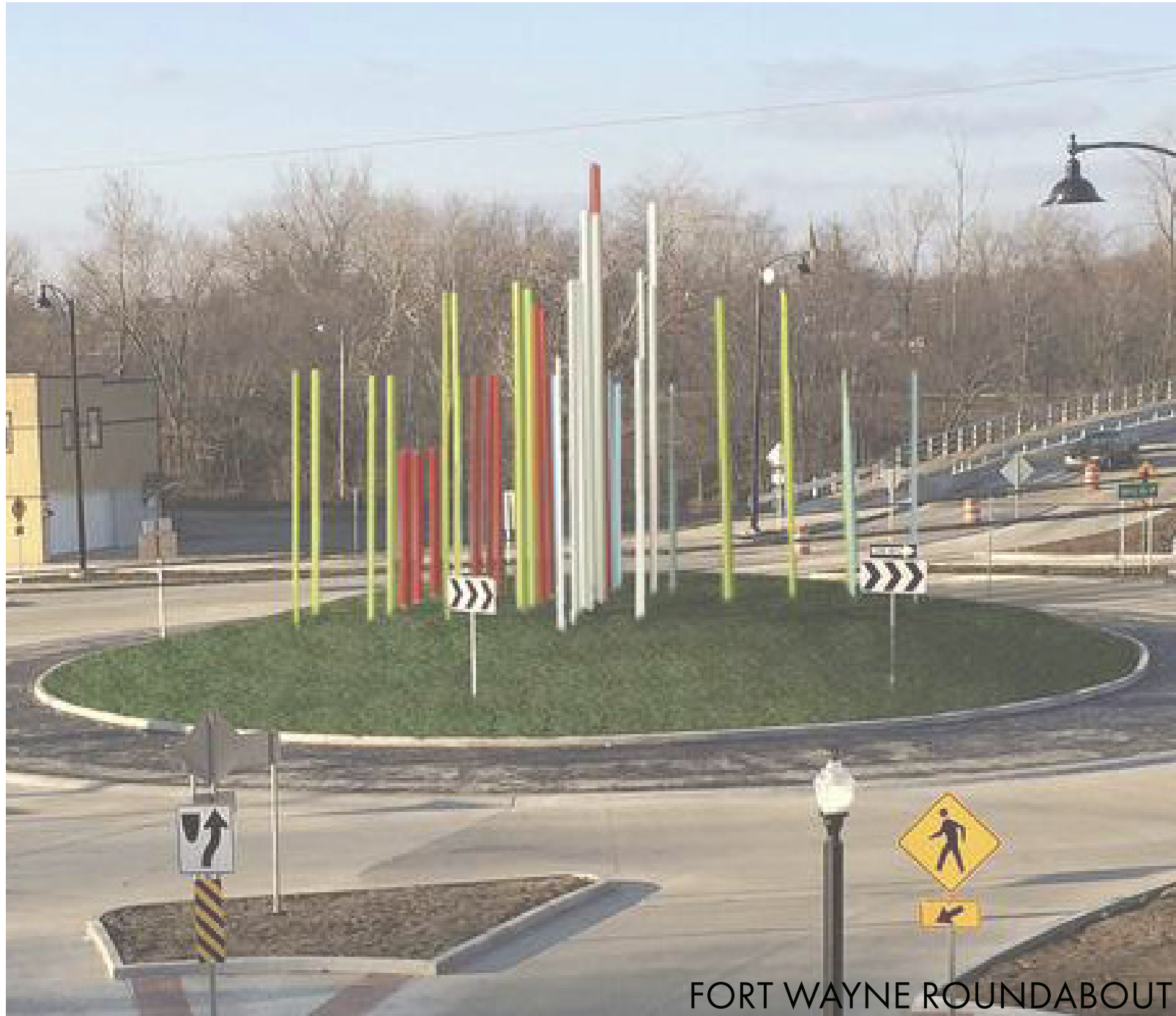
FORT WAYNE ROUNDABOUT
