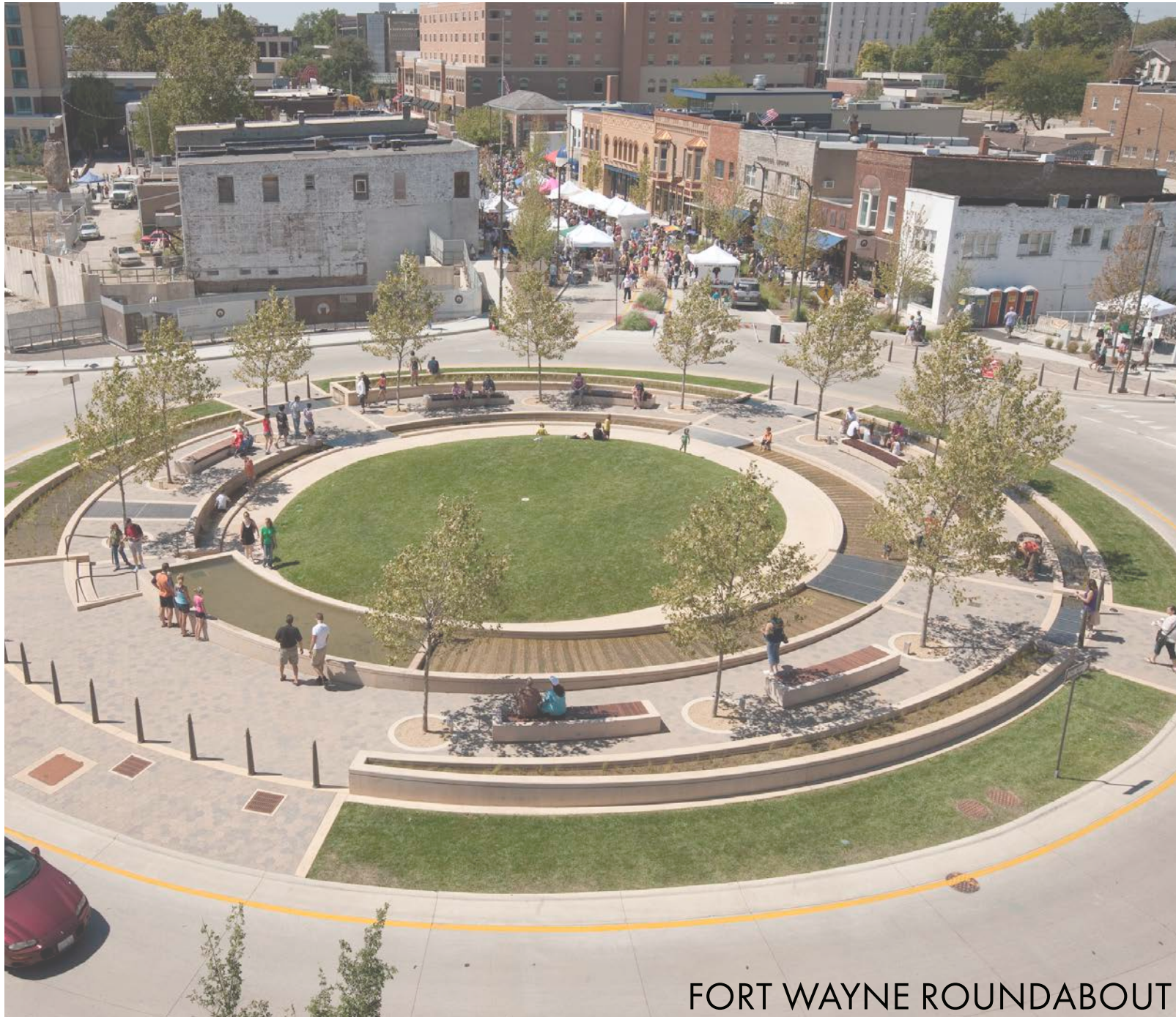
FORT WAYNE ROUNDABOUT
